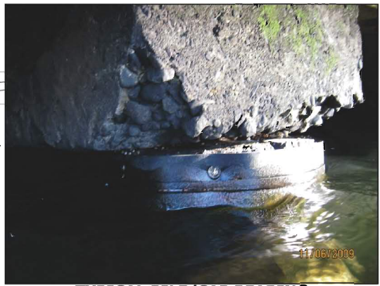
TYPICAL PILE/CAP BEARING
