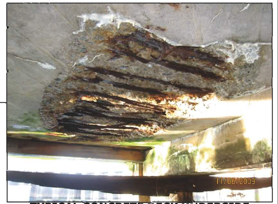
TYPICAL CONCRETE DECK UNDERSIDE
